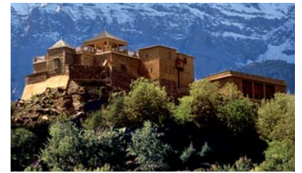
Kasbah du Toubkal, High Atlas Mountains, Morocco: Considerately restored to its former splendour using traditional techniques and local materials, the Kasbah both respects and adds value to the local community. Photograph: Alan Keohane, www.kasbahdutoubkal.com
